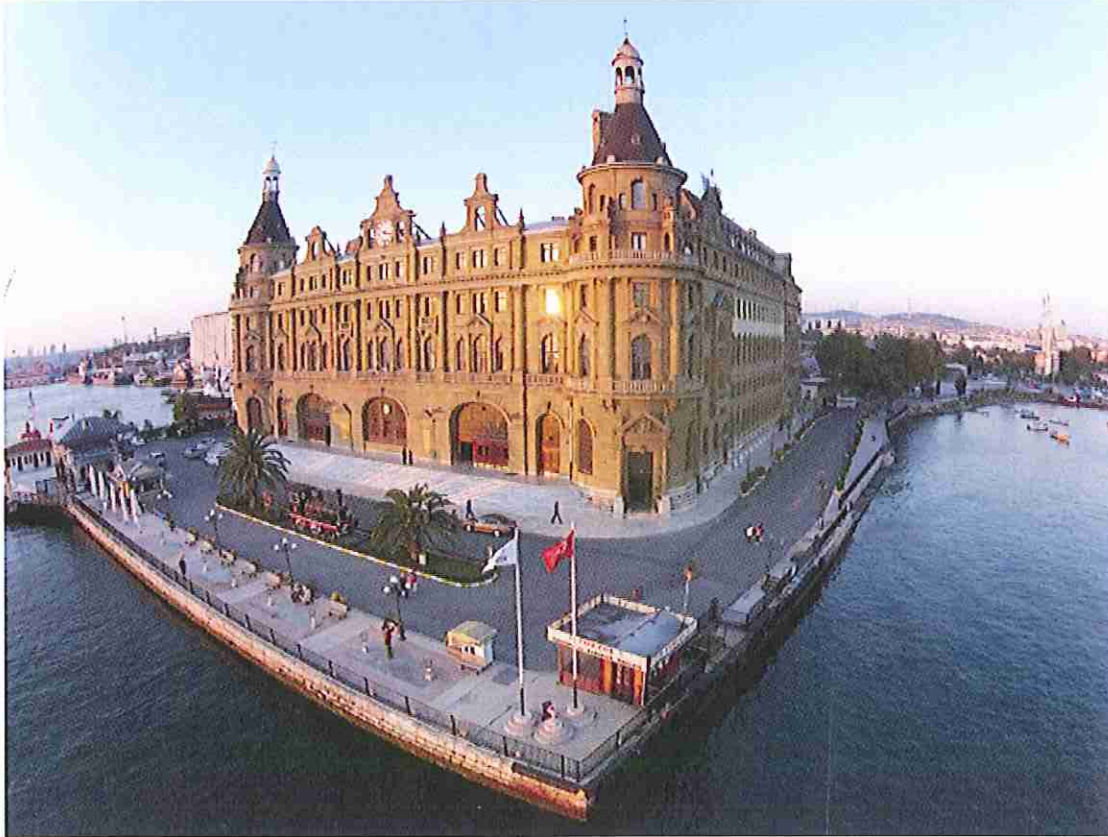
Haydarpaşa Train Station
